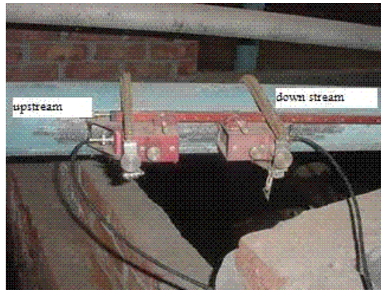
Figure (11): Mounting U-S. flowmeter on steel pipe.
