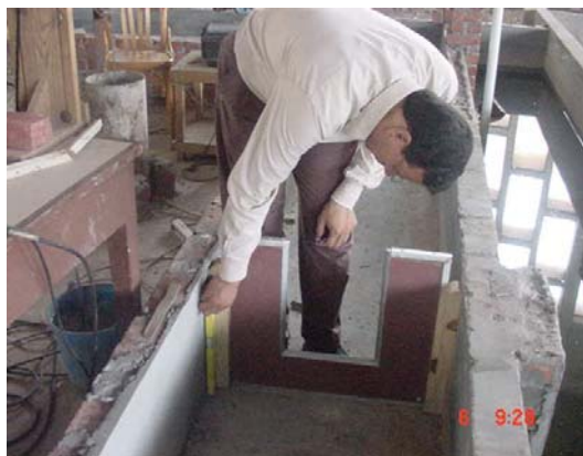
Figure (6): Rectangular weir in vertical direction.
